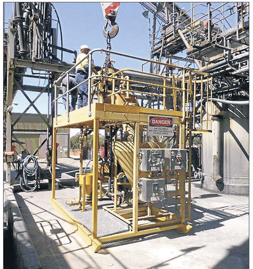
Navarre Minerals' new pilot bulk sample testing facility being relocated into Stawell Gold Mine's mill area.
